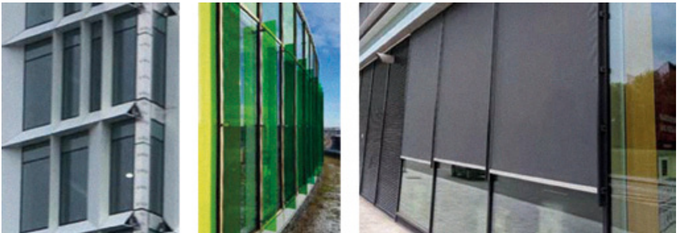
Potential cold bridges caused by fixing of solar shadings and decorative items on facade.
