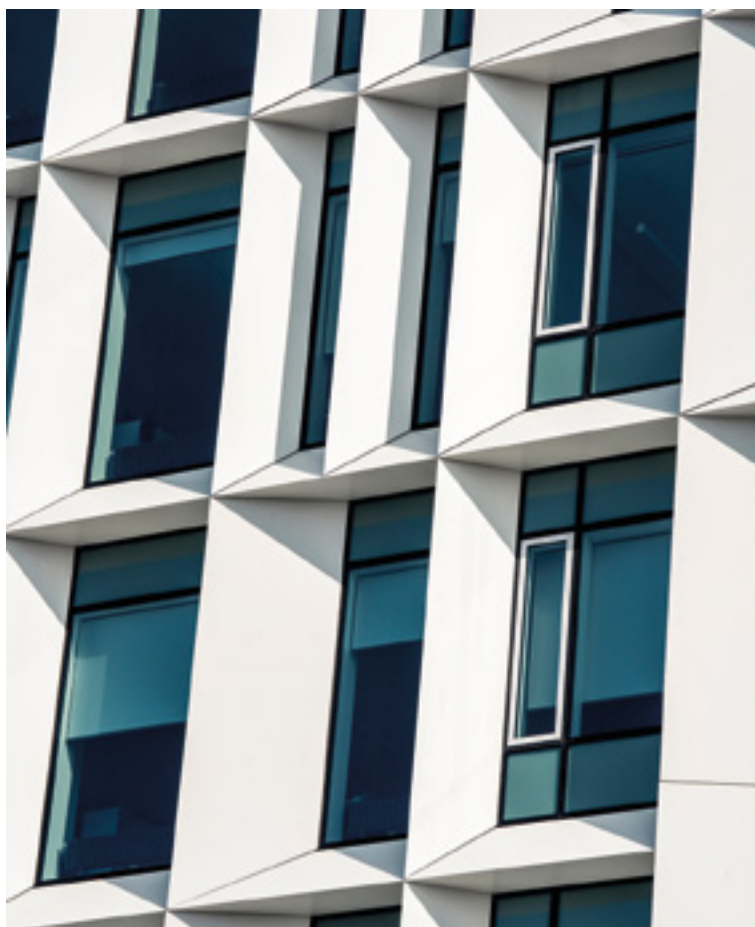
The glass façade is unitized and made with standard products. Every floor has its own carrying structure, so if you want to change the façade in a hundred years that is possible.
